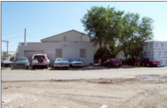
Many of the streets are in poor condition
